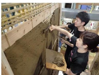
Fig. 4. Plaster of Wall Clay
