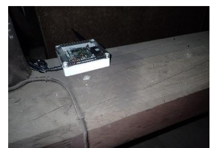
Fig. 6. Installation of Sensor
